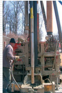
Installation of dilatometer probe
