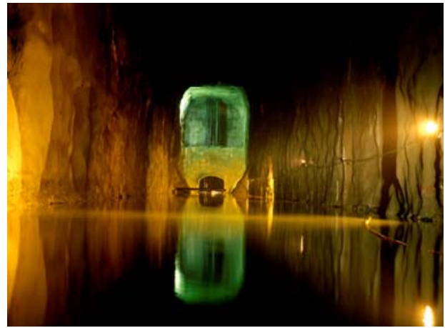
Final cavern shape with changed design due to excess in-situ stresses
