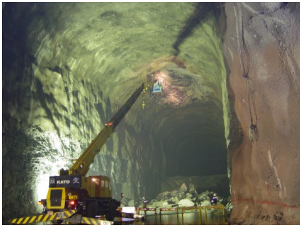
Rock fall treatment in storage cavern
