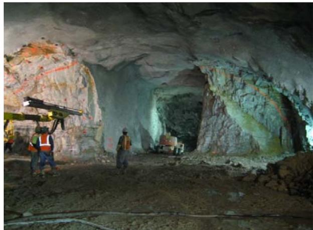
Figure 3: Persistent granitic joint dipping through right side heading.
