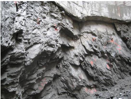
Figure 2: Sub vertical foliation joints of Manhattan Schist as observed in Shaft P.
